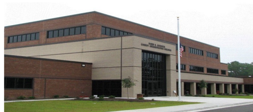
David R. Sandifer County Administration Building
