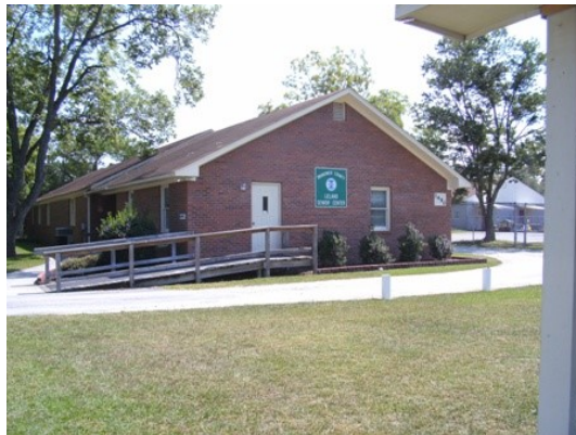
Leland Community Building
